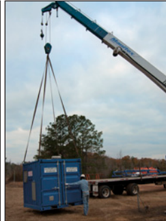
Set Power Unit in Place
