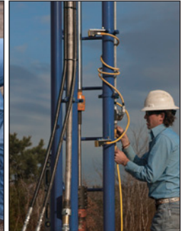
Attach and Adjust Limit Switches
